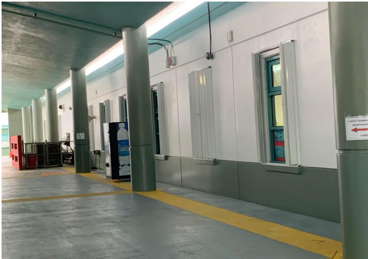
Guam: Window shutters (DOE)
