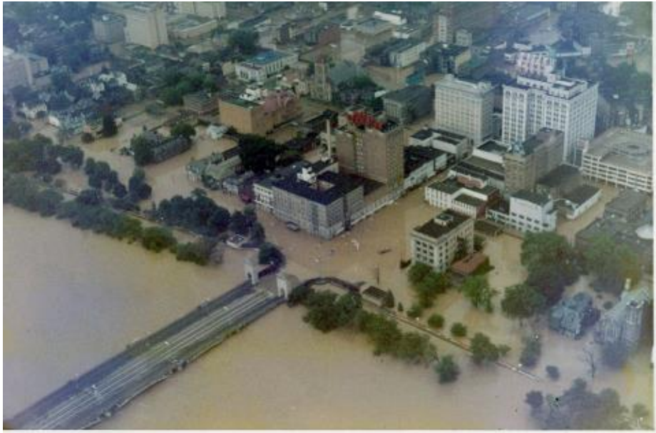
Flooding in Wilkes-Barre, Pa., after Hurricane Agnes, 1972. Office of History.
