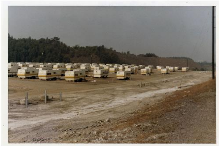
Coal Brook Trailer Park, Pa., after Hurricane Agnes, 1972. Office of History.
