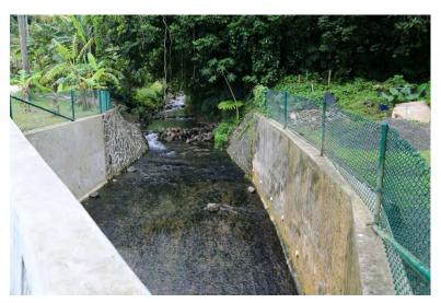
Figure 100 Fagaalu Bridge and Stream Revetment to Protect Hospital.
