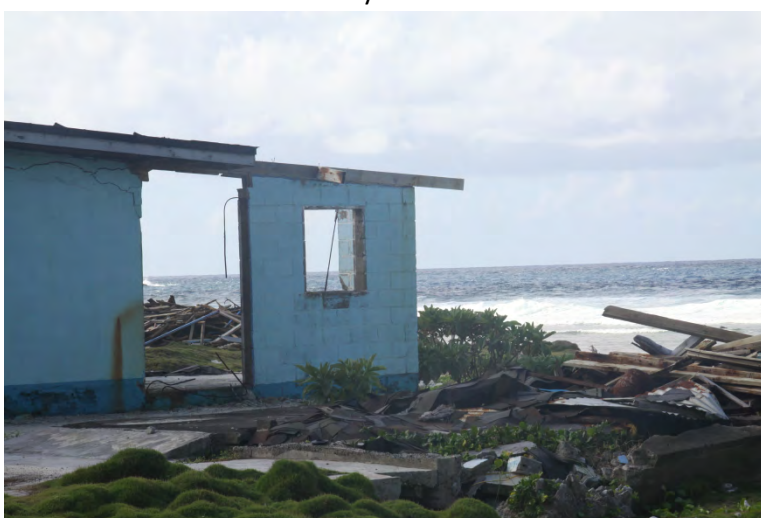
Figure 85: Tsunami Damage from 2010
