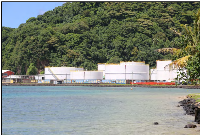
Figure 9 Utulei Tank Farm
