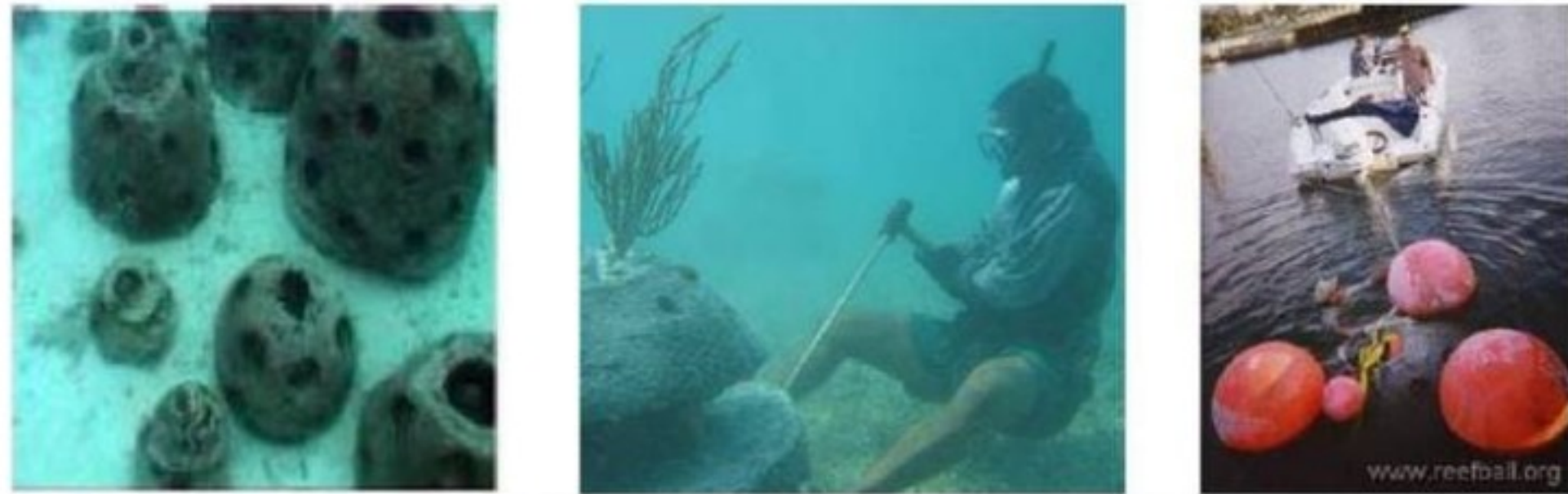
Figure 10-1 - Reef ball installation photos (Reef Ball Foundation, 2018)
