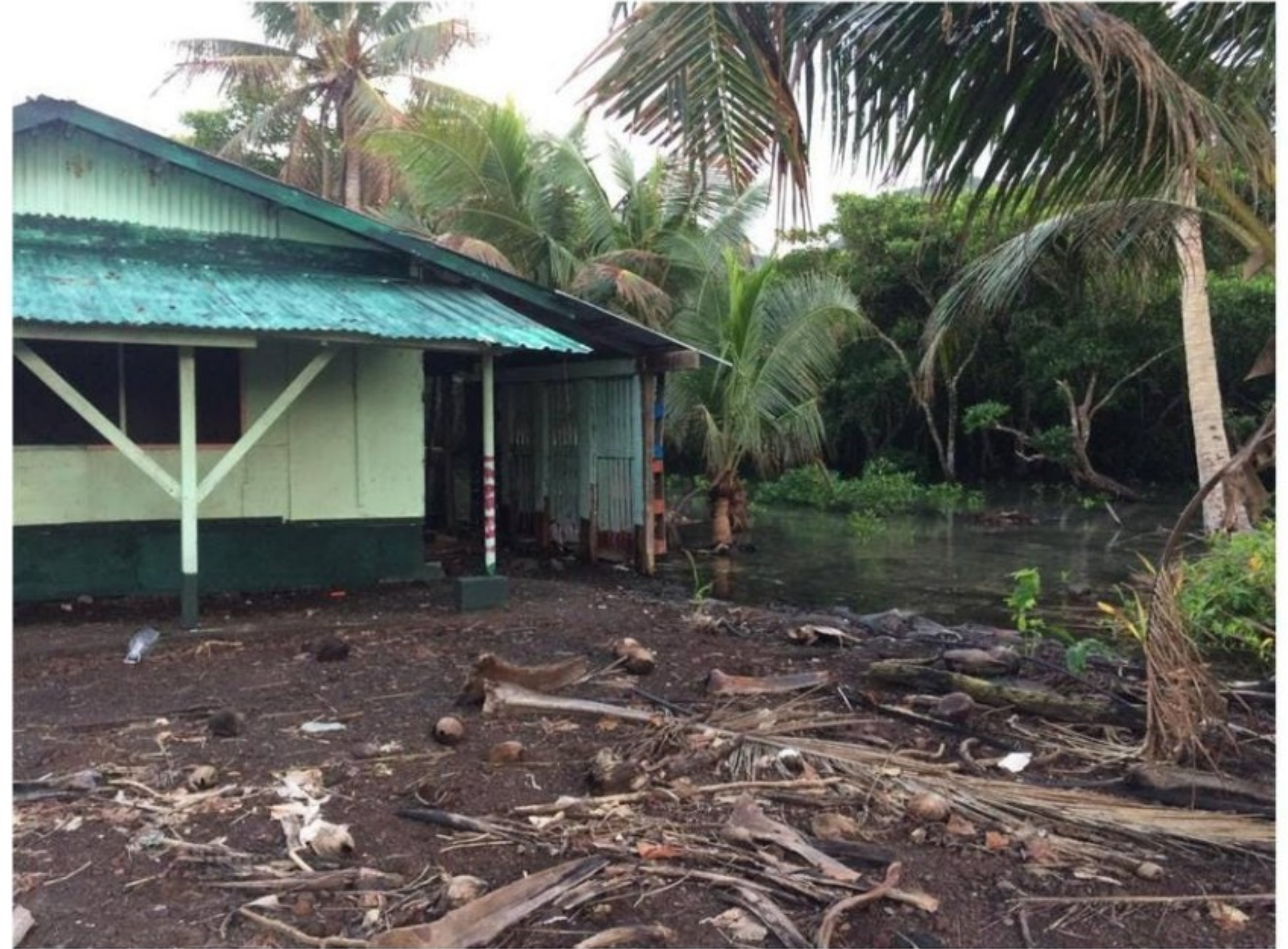
In 2019, Coconut Point, Nu'uuli homes were flooded by a combination of a King Tide event with wind and ocean swell. (Photo by Kelley Anderson Tagarino)
