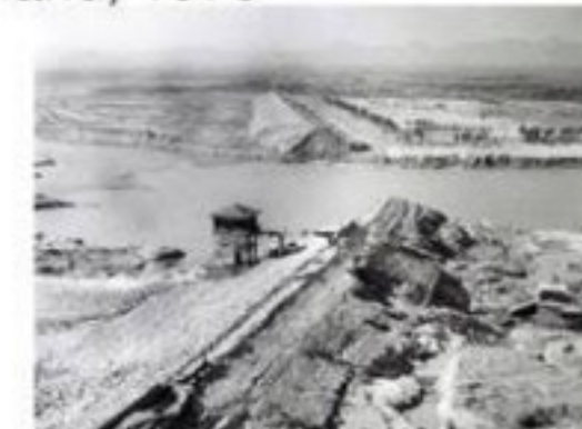
Banqiao dam failure; China, 1975
